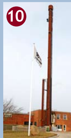
10 VESTERVIG Heating plant (wood chips) Supplies Agger
