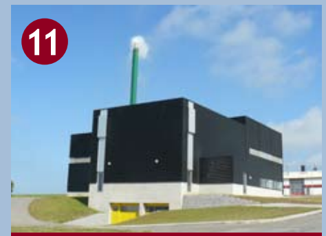
11 HURUP 1: Heating plant (wood chips) 2: Heating plant (wood chips)
