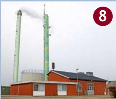
8 SNEDSTED CHP plant (natural gas), 6 MW electric boiler
