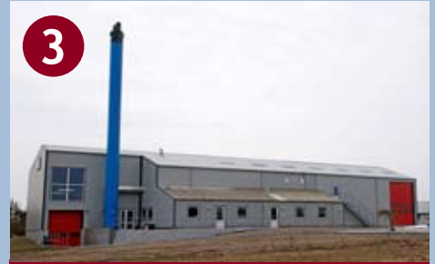
3 ØSTERILD Heating plant (wood chips)
