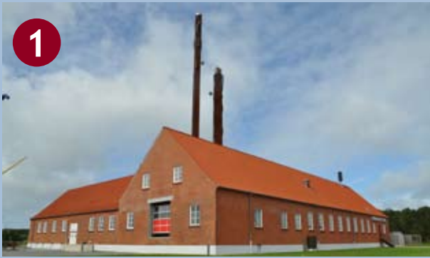
1 HANSTHOLM Hansthholm 1 - heating plant (biomass) Hansthholm 2 - CHP with 10 MW boiler Supplies heat to Ræhr (4.5 km distance)
