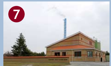
7 VORUPØR CHP plant (natural gas), 1 MW electric boiler
